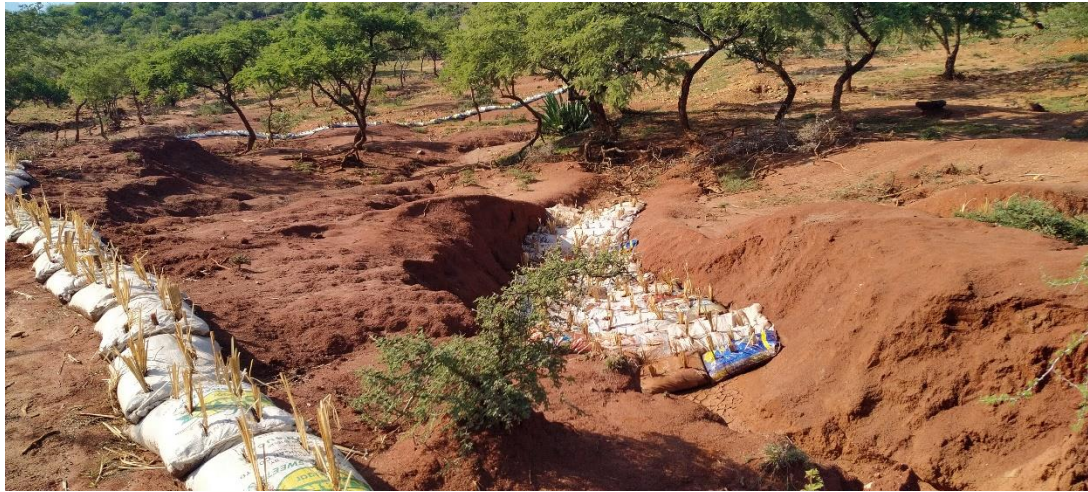
Fig. 9. Vertiver splits planted in the horizontally laid bags along the contour lines and at gully mouth at the Chepareria Livestock Café Annex site (Photos by M Nyaga).
