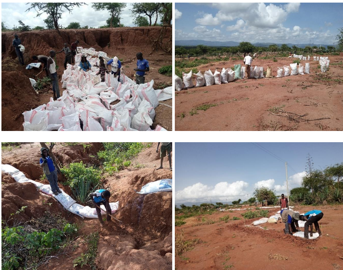
Fig. 6: Filling up of soil bags with the mixtures of sand, soil and manure. Aligning the soil bags along the previously marked contour lines (Photos by M Nyaga).
