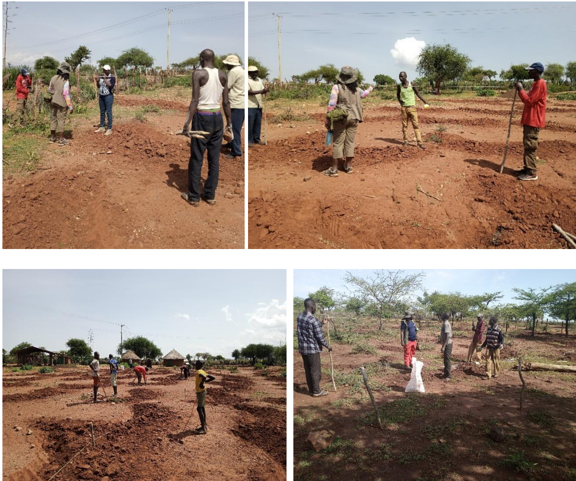
Fig 5: Determining and marking contours using a Line level and White ash (Photos by M Nyaga).
