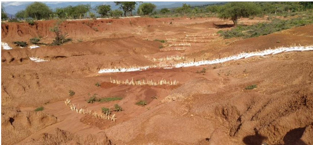
Fig. 8. Vertiver splits planted directly without the bags at the base of the gullies (Photos by M Nyaga).
