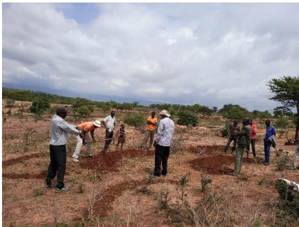
Demonstration on how to dig the trapezoidal bunds. Photo credit: Margeret Nyaga
