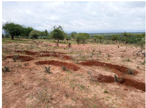
Demonstration on how to dig the trapezoidal bunds. Photo credit: Margeret Nyaga
