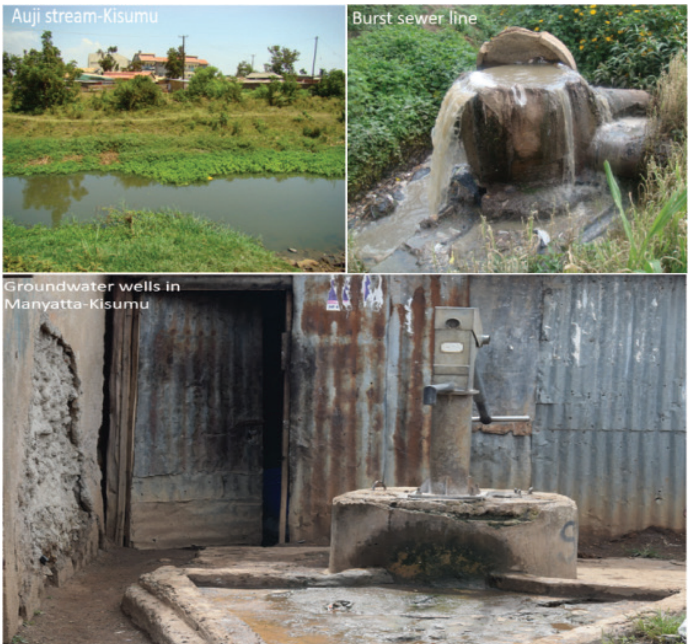
Figure 5. Sewage contaminated streams and burst sewer lines are a major risk to groundwater nitrate pollution especially in Kisumu's informal settlements and in Ahero town.
